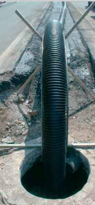
Flexoren system is a renovation method intended for sewer relining. Welded together to cover the entire manhole distance, the Flexoren pipes are inserted in the existing sewer through manholes. The task can be performed principally above the ground with no environmental impact. Flexoren is quick to install and it is the most cost-effective alternative, especially in cases where the line to be renovated is long. Flexoren is also excellent for pipelines with bends.
